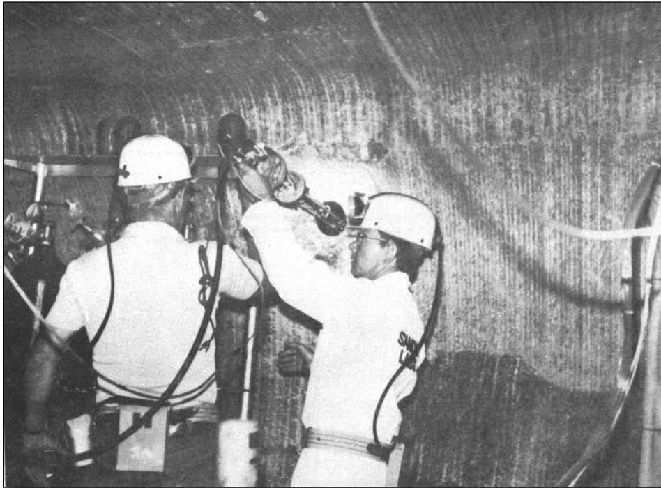
Figure 41. Installation of heater in horizontal borehole at MCC (Figure 5 of Ewing 1981b).
