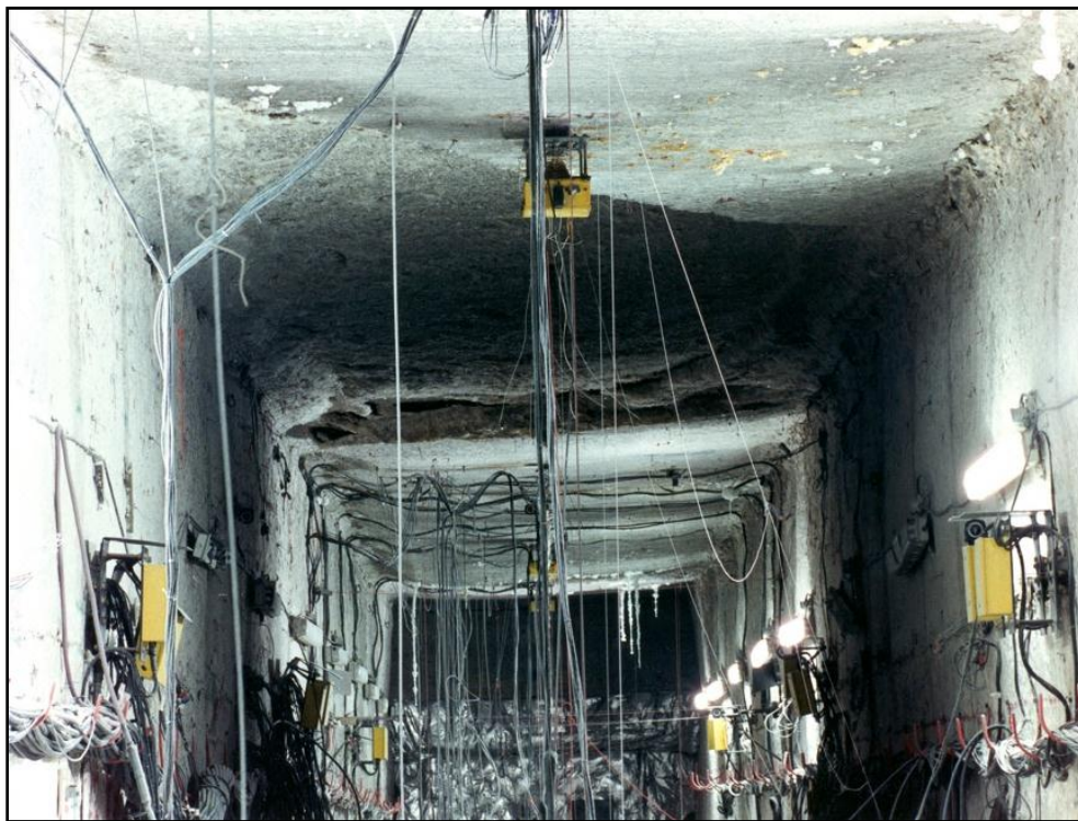
Figure 12. WIPP TSI Room A2 after 1990 roof collapse.
